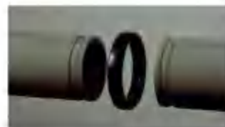
4.Lubricate gasket
